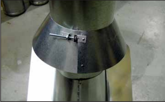
Figure 7.14 - Insert Bolt into Brackets
