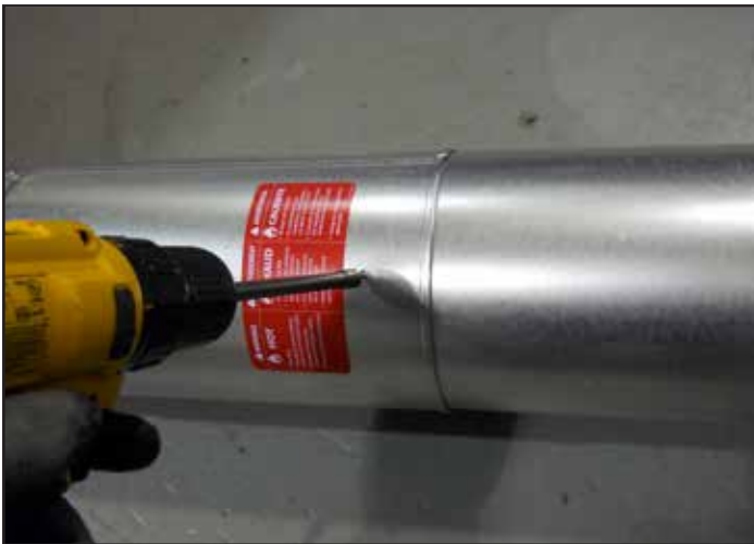
Figure 7.4 - Screws into Slip Section
