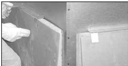
Figure 3.6 Unpacking Back Refractory
