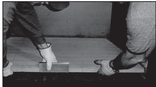
Figure 3.10 Lifting Out Hearth Stone
