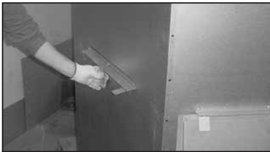
Figure 3.7 Bend Refractory Brackets Back Down
