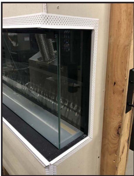
Figure 4.8 Install Appliance
