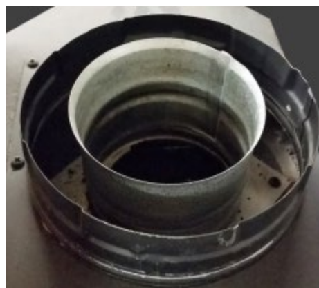
Vent Attachment Inspection – unbent and attached rings
